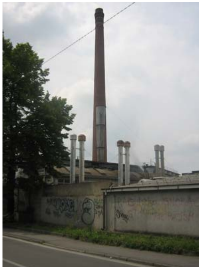
Area Vismara (Casatenovo, estate 2008)
